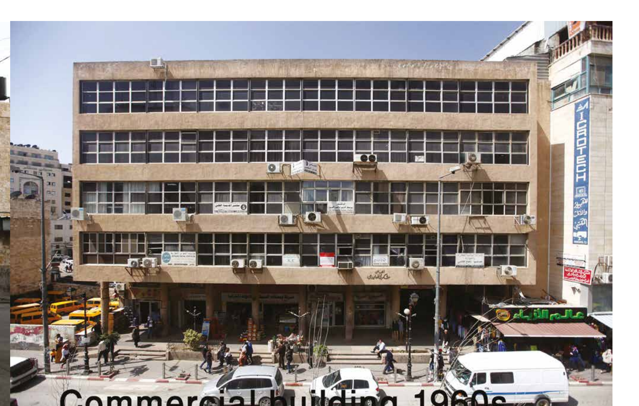
Commercial building 1960s
